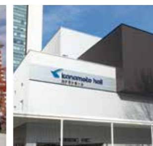
Kanamoto Hall (Sapporo Civic Hall) housing a large 1,500-person event hall as well as small, medium and large conference rooms
