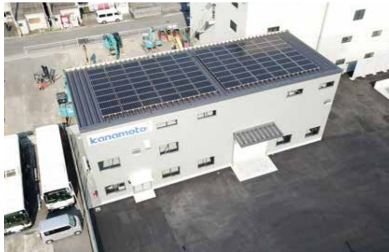
Solar Power Generation System Installed on the Roof of the Kyoto Branch Office
