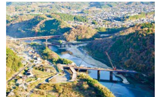
Linear Chuo Shinkansen – Kiso River Bridge No. 1 Construction Project
