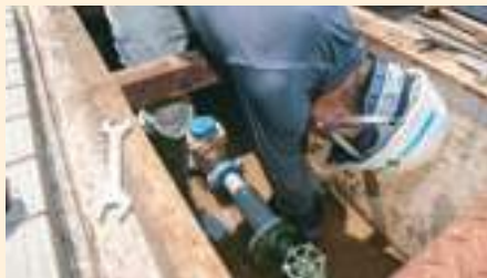
Water Service Connection Point Repair
