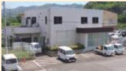
Fukuchiyama Water and Wastewater Service Center
