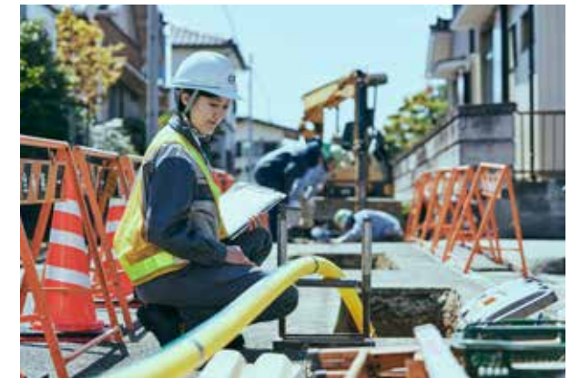
Trenchless pipe installation method
