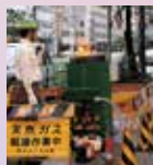
LNG conversion work near Nagoya Station
