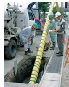
Trenchless pipe installation method
