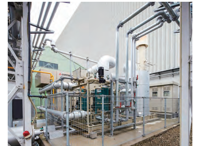
Gas engine cogeneration system
