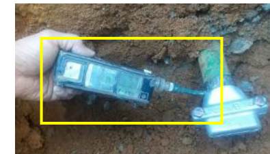
Conducting gas leakage surveys using detectors
