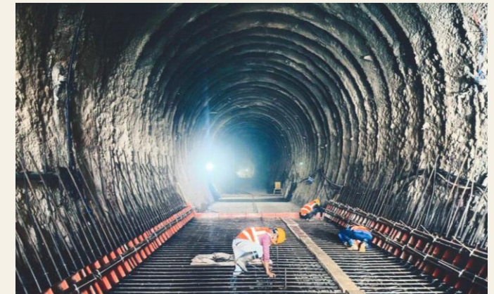
Inside of the headrace tunnel
