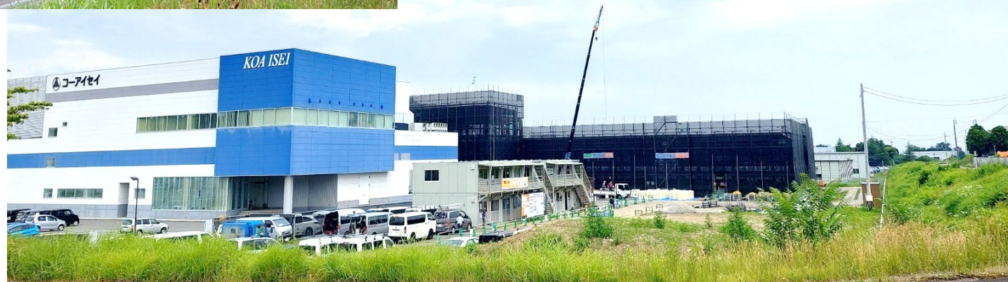
Zao Factory (on the left) and Zao Factory 2 (in the back right)
