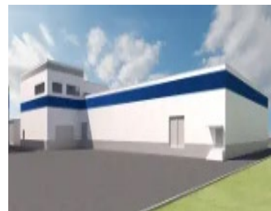
Zao Factory 2 and production equipment
