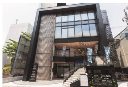
ABENO Well-Being Terrace
