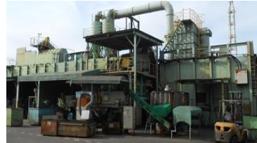
ASR recycling facility (Nishitetsu Metal Co., Ltd.)
