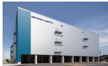
Kanto Logistics Center (Narashino City, Chiba Prefecture)
