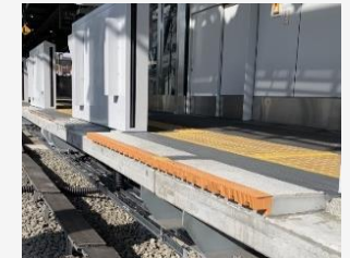
Installation of rubber bumpers for fall prevention Platform elevation
