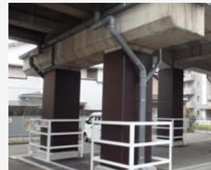
Elevated bridge anti-earthquake strengthening work
