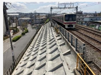
Slope anti-earthquake strengthening work
