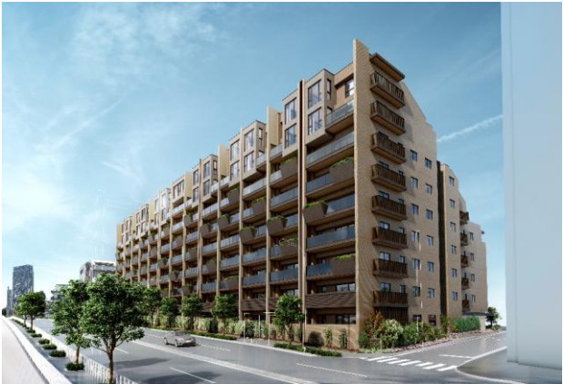
PRIME Yokohama (Hills)
