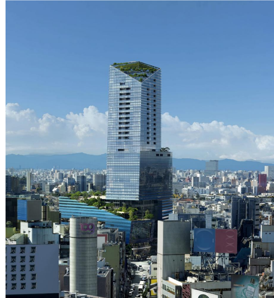
Shibuya Upper West Project Façade image Image by Mir / Copyright : Snøhetta and NIKKEN SEKKEI LTD
