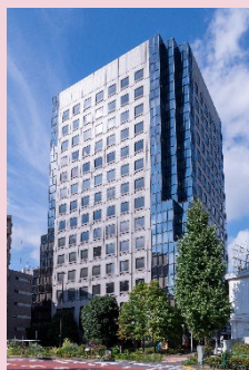
Osaki MT Building
