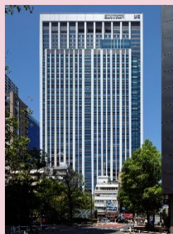
Kamiyacho Trust Tower
