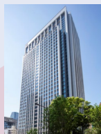
Kamiyacho Trust Tower
