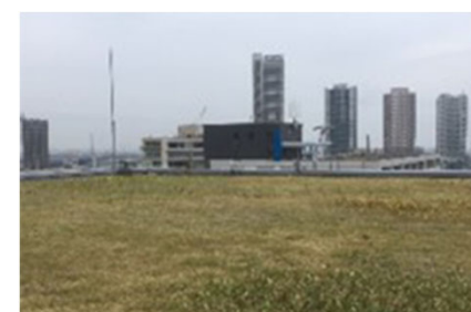
Toyosu Prime Square (Rooftop)
