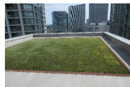
Yokohama Plaza Building (Rooftop)
