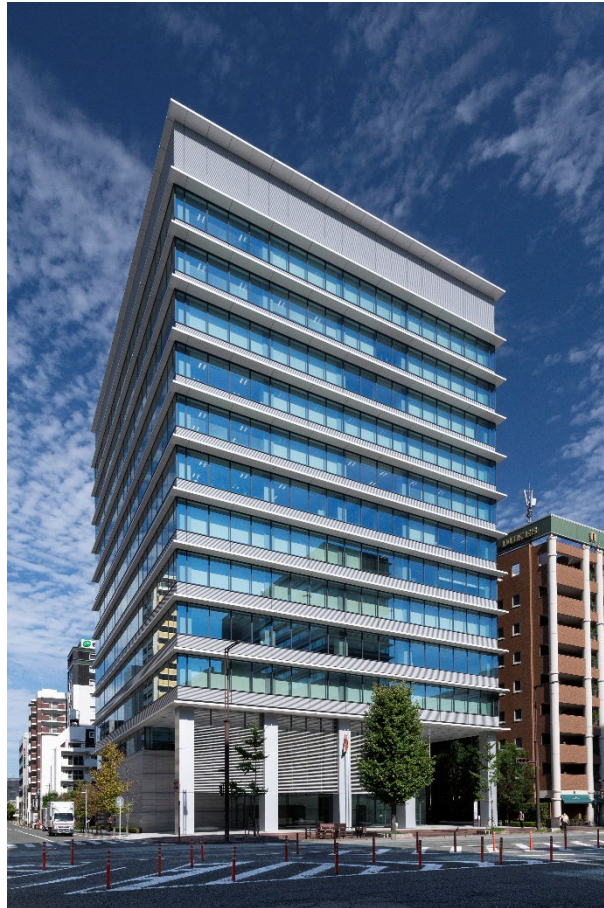
<Ref. 1> FUKUOKA K-SQUARE: Building photo and access
