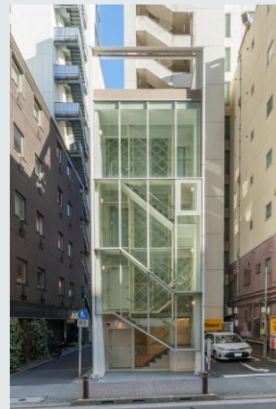
Ginza SLC Building
