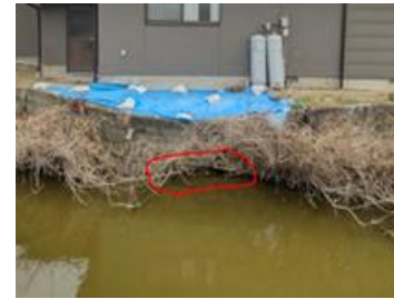
A case where residential land damage caused by erosion from a nearby waterway was discovered after sale. Significant costs were incurred for erosion control measures.
