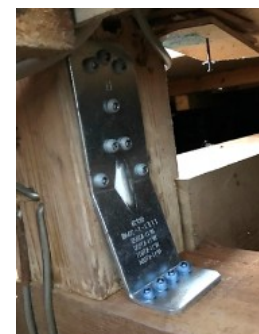
Installation of seismic reinforcement fixtures
