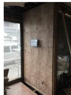
Installation of new earthquake-resistant walls
