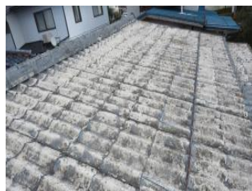
Case in which deterioration in roof materials was noticed after sale. As a partial repair was not possible, the entire roof had to be replaced.
