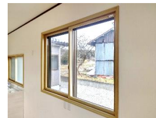
Example of installing double-paned window
