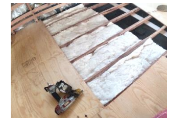
Example of installing insulation
