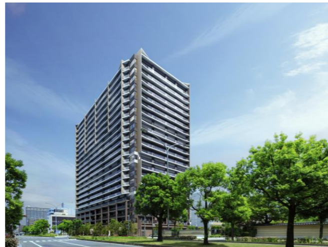
Sendai THE GRAND SKY (Joint venture total Units 476 units)
