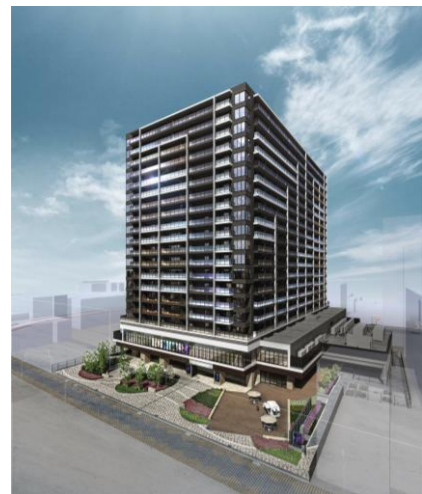
LEBEN Odawara SKYS THE TOWER (Joint venture total Units 286 units)
