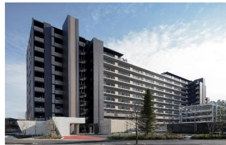
Kawagoe Nandai Rebuilding Project
