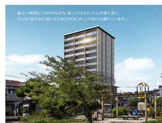
Branneed Kawachieiwa 13F 38 residence RC building (Completed on May 17, 2024)
