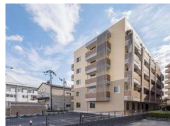
Ikyu Esaka 68-room steel structure (Completed on February 18, 2022)
