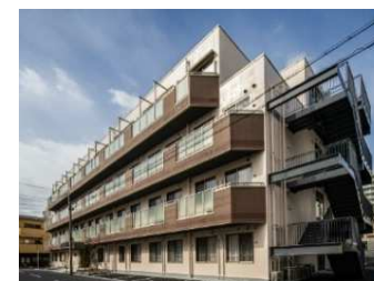
Hibio Sumiyoshi 78 rooms (former hospital) (Completed on February 3, 2025)
