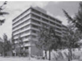
Keihanshin Kawaramachi Building (Completed in 1962)
