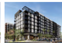
Jefferson Portico Project (for-rent condominiums)
