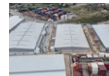
Laem Chabang Project (logistics)
