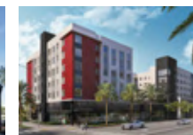
Campanile at SDSU Project (for-rent condominiums)
