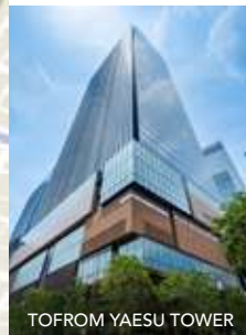
TOFROM YAESU TOWER
