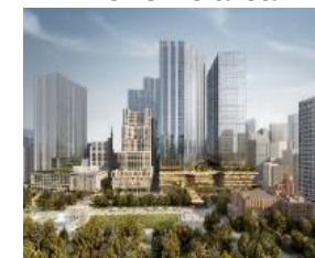
South block (South Tower)
