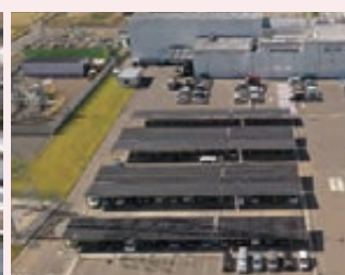
Solar panels at Aoki Foods
