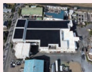
Solar panels at Akune Plant
