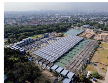
La Mesa Water Treatment Plant (Philippines)
