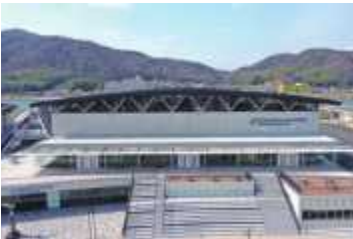
FPCO Arena Fukuyama
