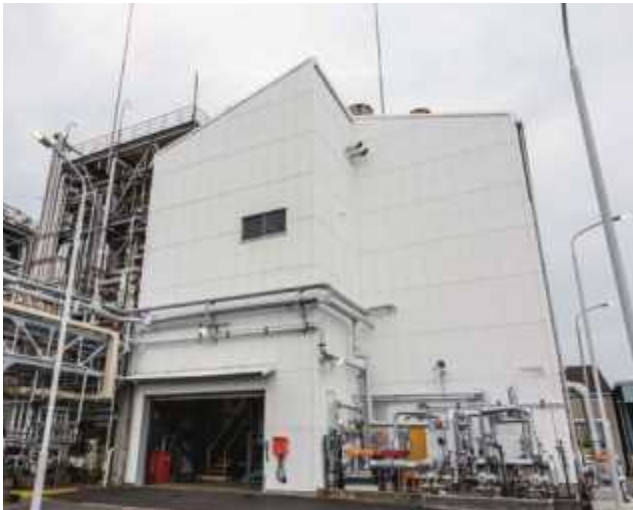
A facility for deinking colored pellets (the materials used to make trays) using dissolution and separation recycling technologies constructed at DIC's Yokkaichi Plant
