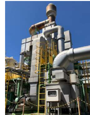
Exhaust gas treatment system at the Numazu Plant
