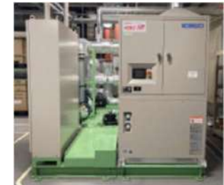
The waste heat recovery heat pumps at the South Plant of the Numazu Plant
