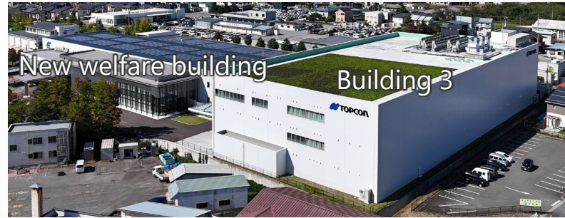
Together with the current buildings 1 and 2, production capacity will be increased by 50%*
