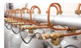
Gas-based fire extinguishing systems are useful in facilities where water and foam extinguishing is not suitable, such as factories, office buildings, museums, and multi-story parking garages.
