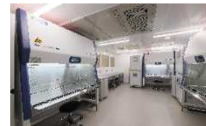
Construction Example) CPC cell processing facility
