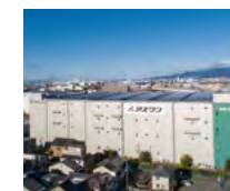
Hanshin distribution center (Amagasaki)
