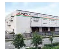
Osaka Logistics Center
