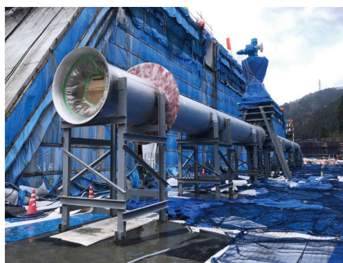
Asuwagawa Dam hydraulic gate equipment for the Kinki Regional Development Bureau (water level adjustment discharge pipe and gate equipment)
