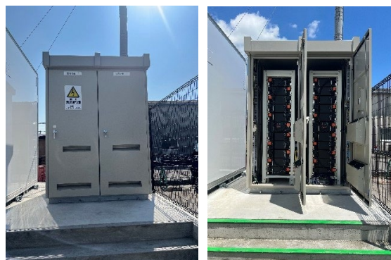
Lithium iron phosphate ion battery unit for the Ogi City Hall off-grid system in Saga Prefecture
