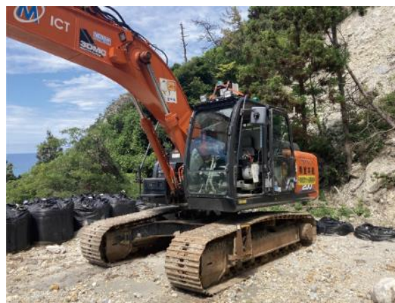
Construction machinery for 3D remote operation (Wajima City, Ishikawa)
