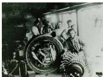
Repairing electrical machinery
