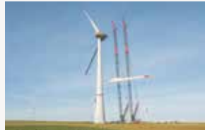
Assembling wind power generation equipment
