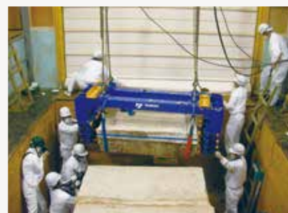
Disassembly of the Takamatsuzuka Tomb's stone chamber
