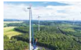
Assembling wind power generation equipment
