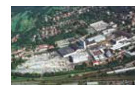
TDG (Germany): Dinglerstraße Plant
