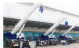
Paint shop at the Shido Plant
