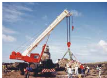
Moai Statue Restoration Project
