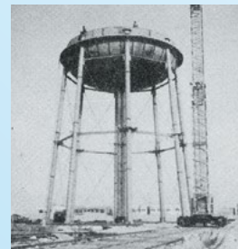
Elevated water tank under construction in Kuwait
