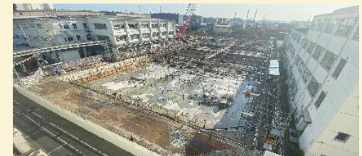
Situation as of April 2026: Reinforcement bar assembly process
