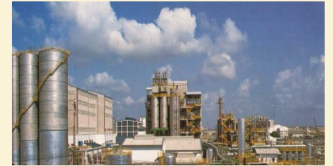
Plant construction example
