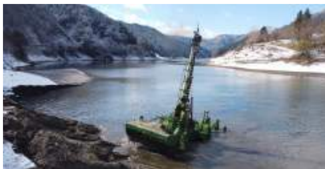
Amphibious bulldozer performing dredging work at a dam
