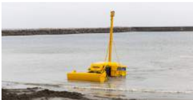
Underwater construction robot concept machine testing at a port
