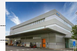
New NP Building
