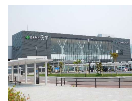
JR Hokkaido Shin-Hakodate-Hokuto Station.
