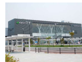
JR Hokkaido Shin-Hakodate-Hokuto Station.
