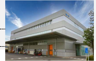
New NP Building
