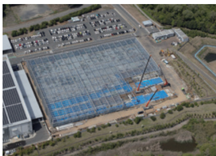
Shimotsuma Warehouse (Shimotsuma City, Ibaraki Prefecture)
