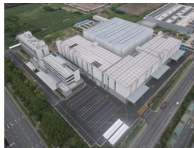
SMC China, Changzhou Warehouse (Changzhou)
