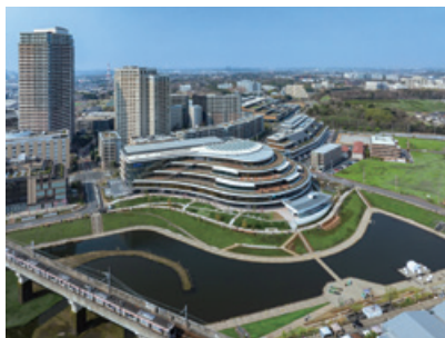
Japan Technical Center (Kashiwa City, Chiba Prefecture)
