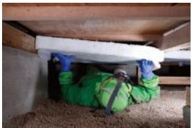
Underfloor Insulation
