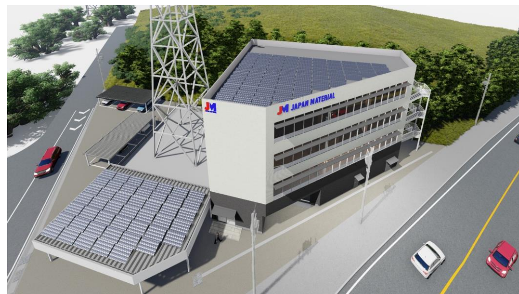
Yokkaichi Branch under reconstruction
