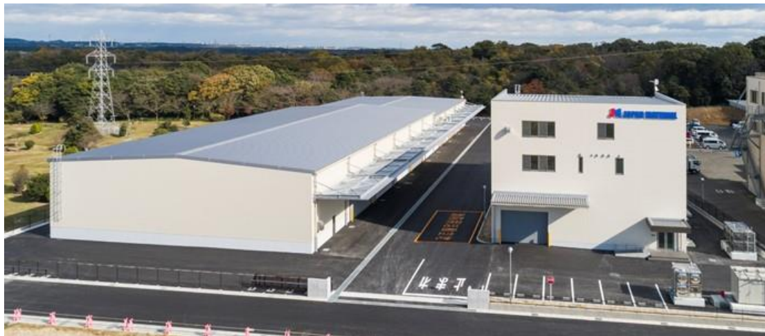
Technical Support Center (left: warehouse building; right: technical building)
