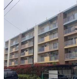
Apartment exterior wall repair work (Building Renewal)
