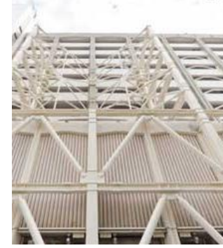
Apartment building earthquake resistance reinforcement work (Building Renewal)
