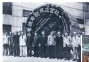
Shipment of high-voltage cables (Photographed in 1939)
